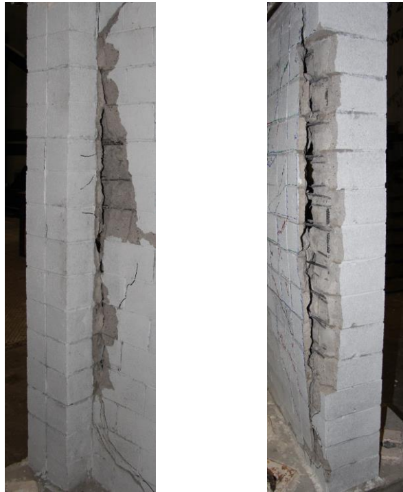
Fig 3.9. BEs-Web connection failure of Wall 5
