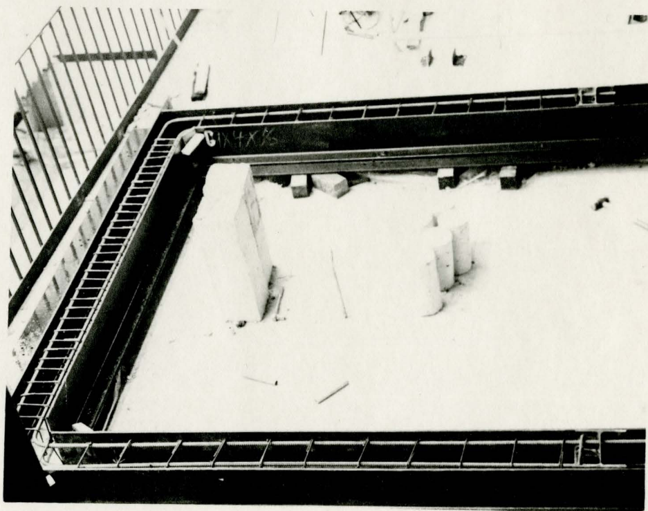
FIGURE 3.3. REINFORCING CAGE
