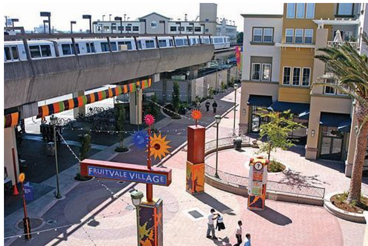
Figure (6-4). The completed Fruitvale Transit Village in Oakland includes a mix of affordable housing, community services and retail space. It is connected to Fruitvale's commercial center via a popular pedestrian-only plaza. (Source: Chapple, Hickey, and Rao, 2007)
