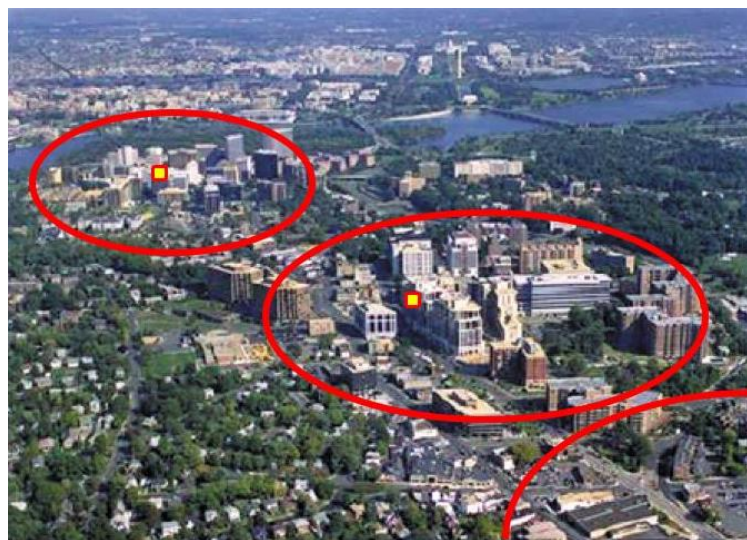
Figure (6-2) Applying TOD on a metropolitan scale to reshape Rosslyn-Ballston transit corridor in Arlington, Virginia. High density, mixed use development is concentrated within 1/4-1/2 mile from stations (shown in red), with limited density outside those areas. (source:Wikipedia.com)
