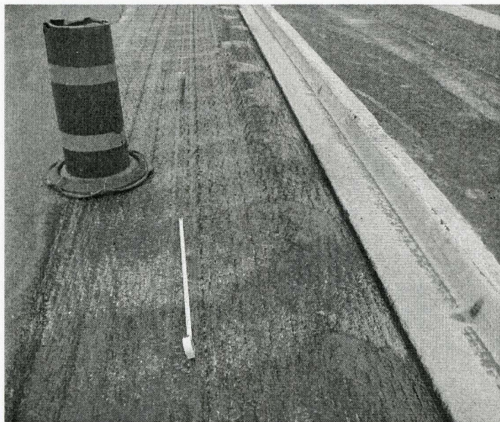
Figure 6-7: Section of the Traffic Lane Marked for Testing (Prior to Paving).
