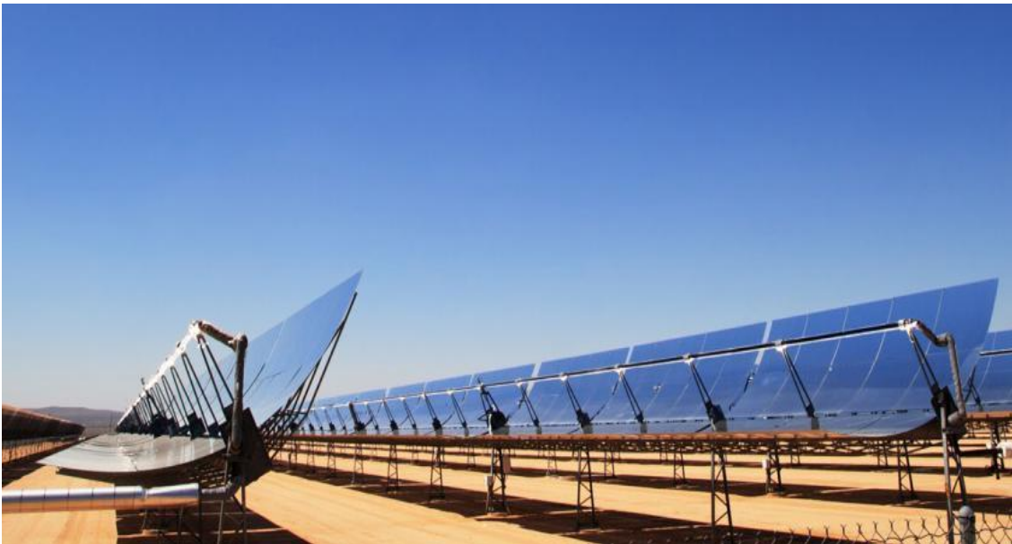
Figure 1.3: Solar energy harvesting using concentrating solar power technology [3].
