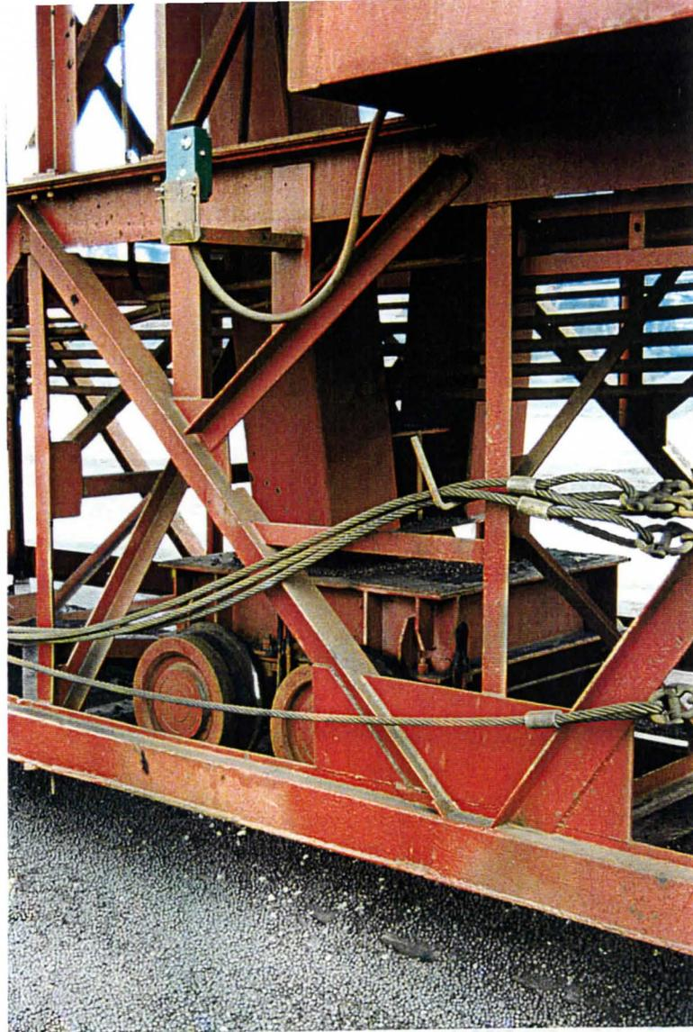
**FIGURE 59:** View of the south hopper truck within the sill truss.
