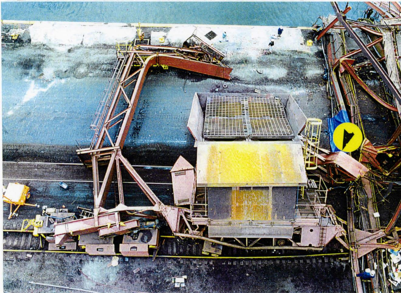
**FIGURE 11:** Aerial view of North Leg of Shear Leg and hopper (looking east). (Arrow points to haunch section) (Dofasco, 1995)
