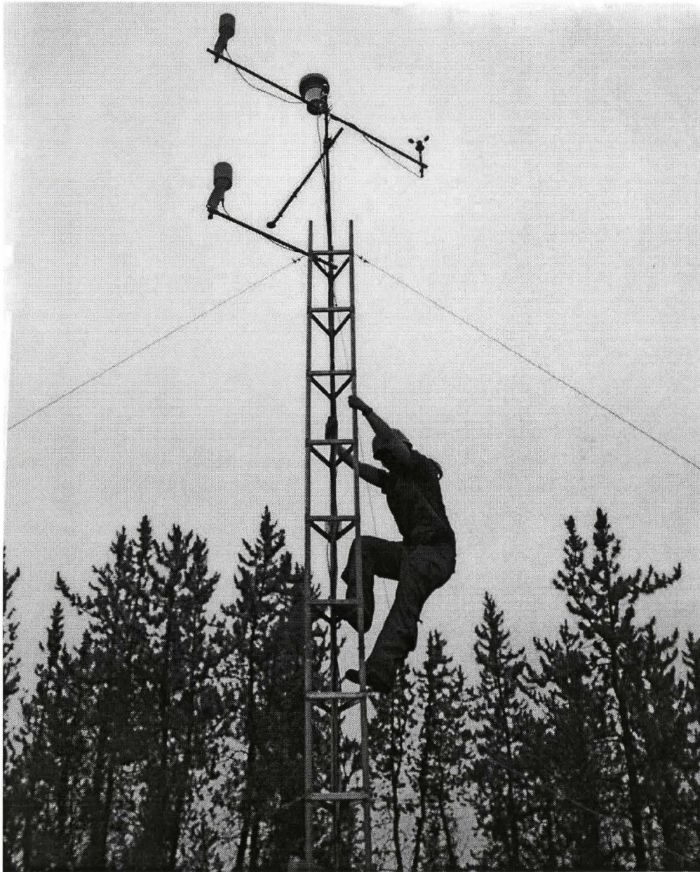
Figure 3.3: The upper section of the soil-filled bottomland climate tower showing instrument deployment.
