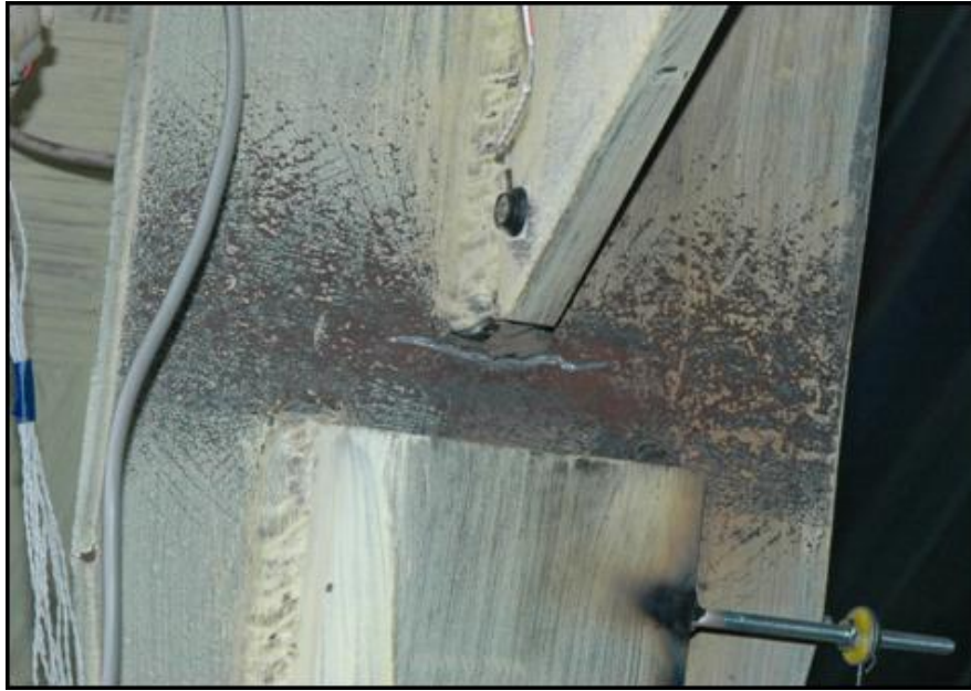
Figure 1.10: Knife plate damage with insufficient hinge clearance (Lumpkin 2009)
