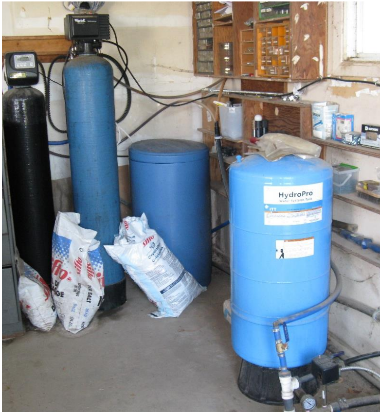
Figure 3.1: A typical treatment system for a domestic well sampled as a part of this study. Untreated groundwater was always collected, often from the base of the pressure tank.
