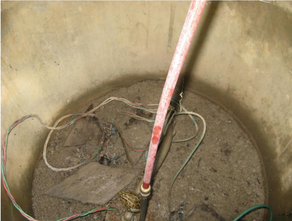
Figure 3.3: An unsecure well in a well pit. Signs of water damage from flooding is apparent on the sides of the well pit. Well locations were determined using a global positioning system device and transferred into geographic information software (ESRI®ArcGIS®). 120 samples were collected in the summer of 2015 from domestic and farm wells and 7 samples were collected from several groundwater-fed springs. 29 monitoring wells were sampled in the study area using consistent sample collection protocols. 26 additional quality-control samples (blanks, standards and duplicates) were submitted with the collected samples for laboratory analyses, for a total of 182 samples.
