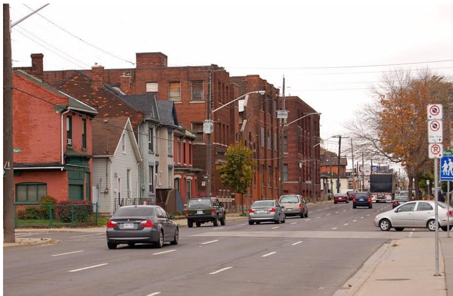
Figure 2.1 Before a Separated Bike Lane on Cannon Street, Hamilton.
