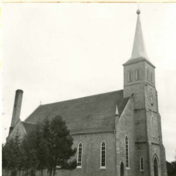
Photo 63. The Roman Catholic Church, the centre of the village's religious life. The structure cost $50,000 to build in the 1870's.
