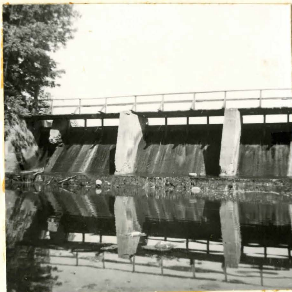
Photo 53. The dam on the Teeswater River at Little's Mill. The mill uses water power almost exclusively, relying only on auxiliary diesel power when necessary.
