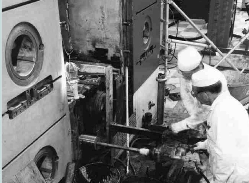
When the DUALSPEC instrument was installed in the early 1990s some modifications were made to the main concrete shielding of the NRU reactor.
