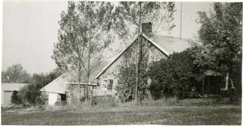
No. 43. The unshaped field stones in the masonry contrast with the large, skilfully squared stones of the house above. Con. II
