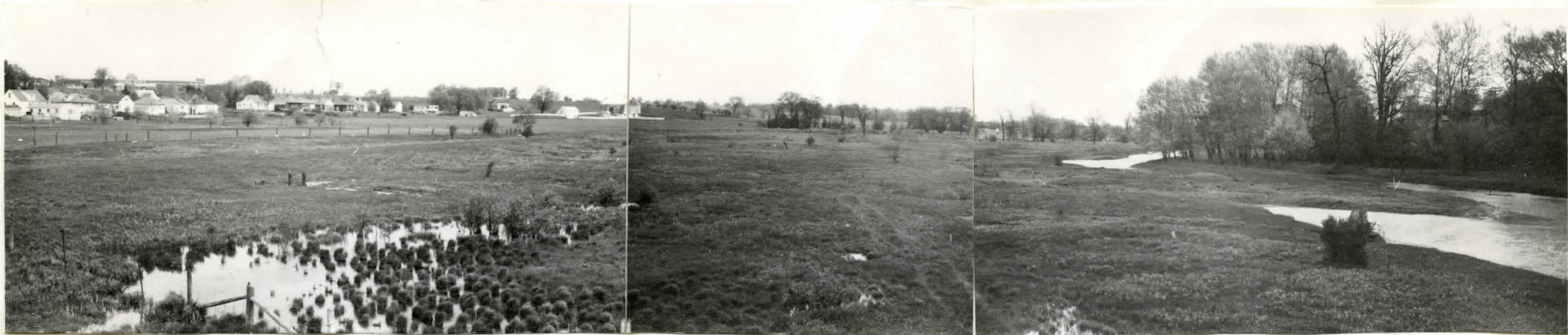
No. 24. The Thames spillway at Woodstock. View to the North. The projected Woodstock reservoir will be constructed further upstream.
