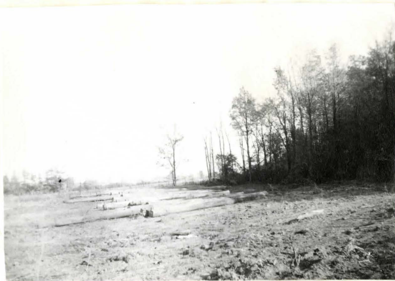
No. 49. Forest edge cleared for tillage. Land to be tile drained before cropping. Hardwood logs destined for sawmill. Con. XIII
