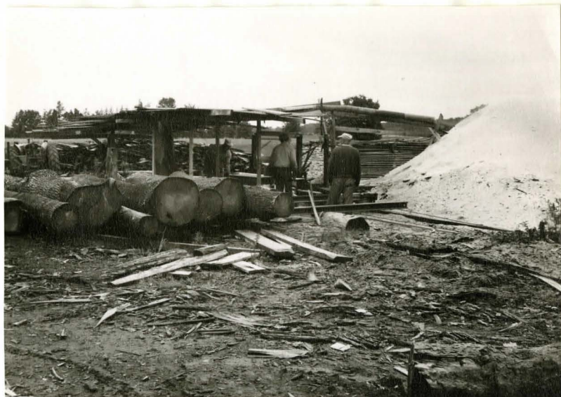
No. 50. Sawmill close to Highway No. 2 draws logs from several townships. Maple, white ash, bass wood, red oak, cherry, elm are among the hardwoods sawn into lumber for export.
