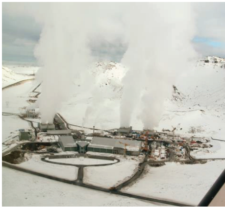
Figure 2.4.2: Hellisheiði Geothermal plant in Reykjavik, Iceland.
