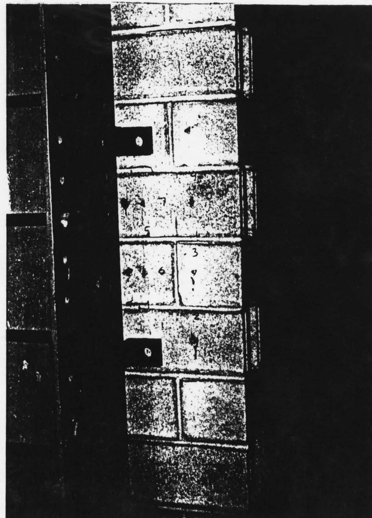
Fig.4.6 Tensile Side of Wall P2 after Failure.
