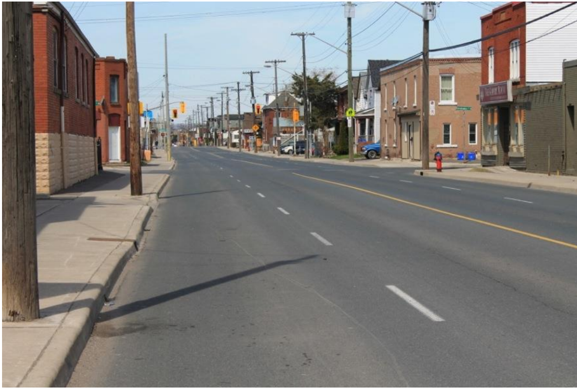
Figure 4-6. Cannon Street East near Gage Avenue North
