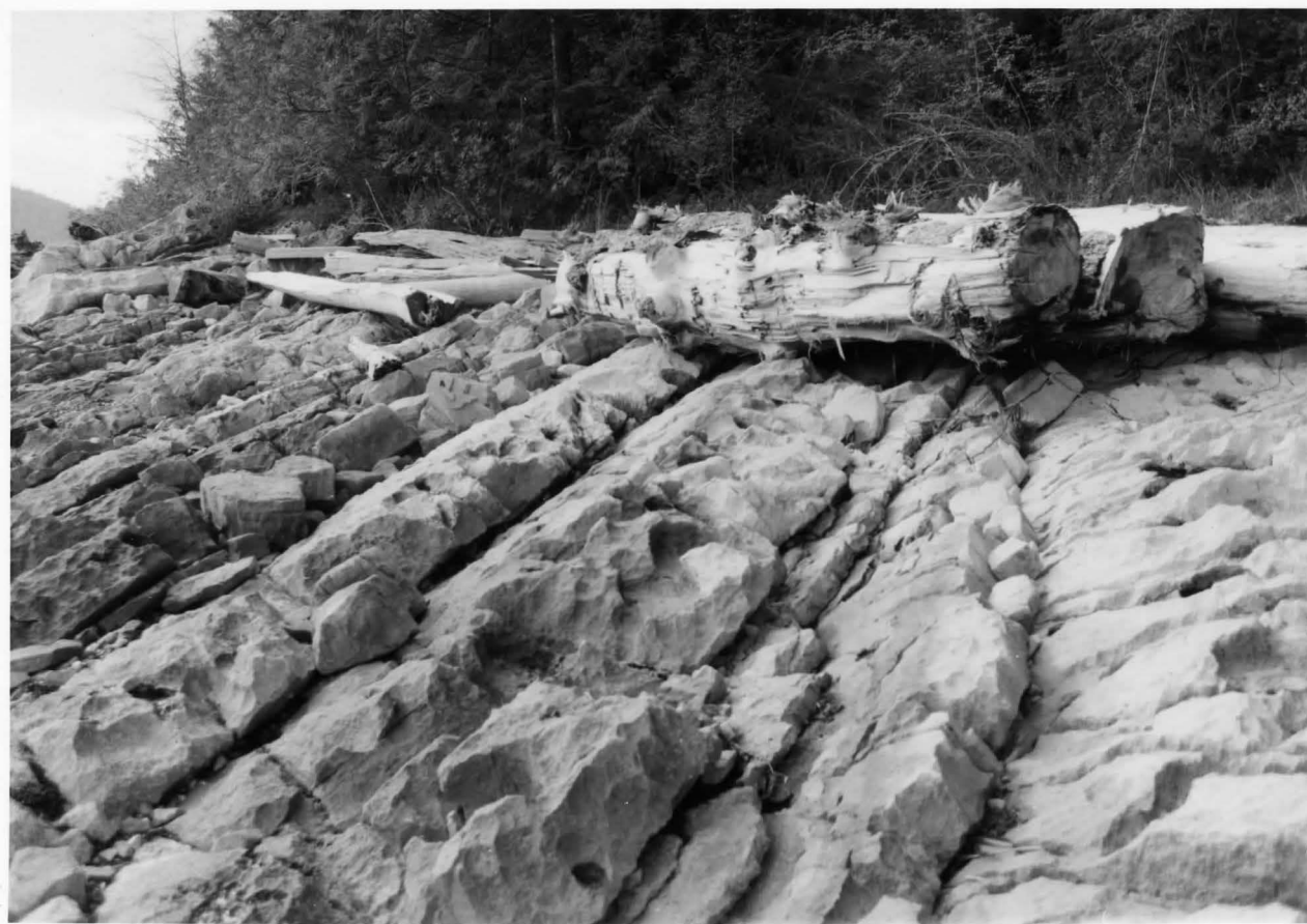
Figure 3.5 Typical High Tide Scene: Dominated by Large Pits and Fractures
