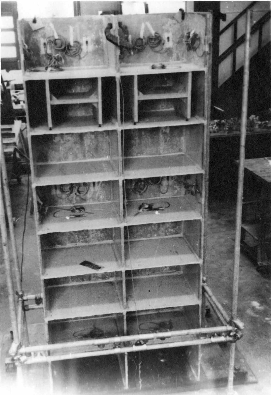
PLATE 1 INSTALLATION OF THE LAST LEVEL OF FLOOR SLABS IN BUILDING 1
