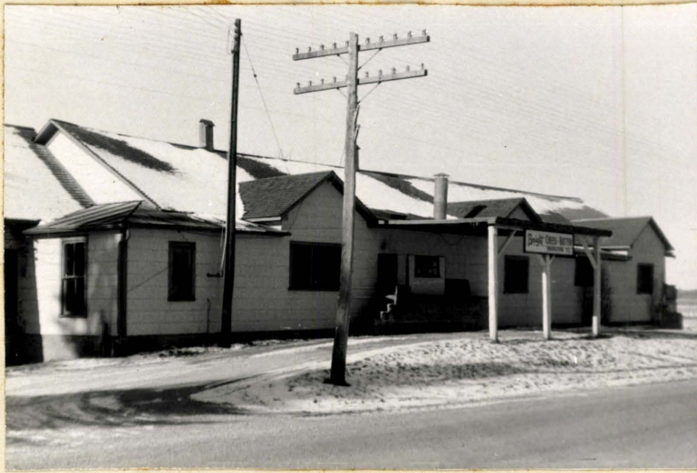
Fig. 22. Bright Cheese-Butter Mfg. Co. located on the northern outskirts of Bright. Much of the milk from N.W. Blenheim Township is sent to this plant.
