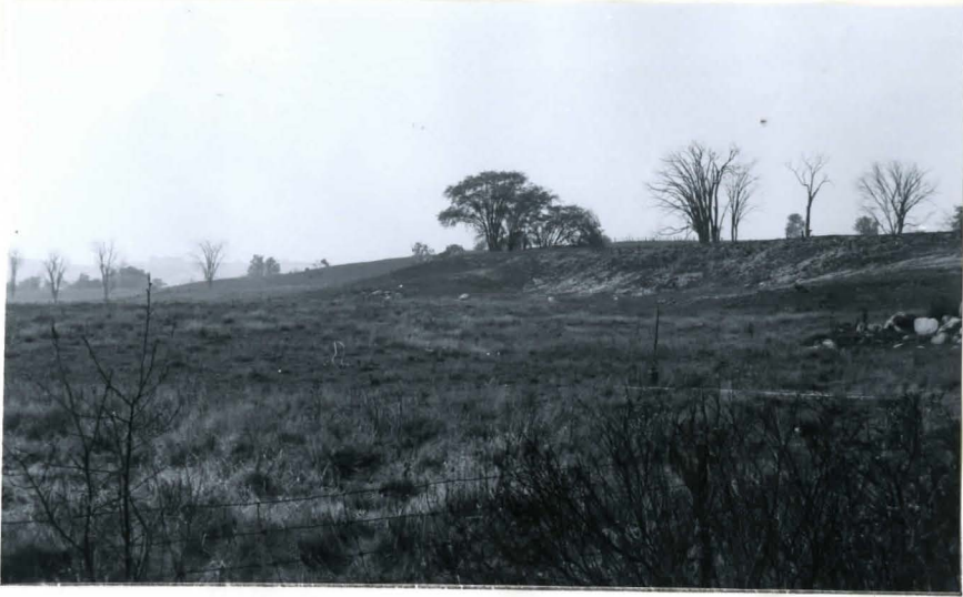
Photo. 5-92 Iroquois coastal bluff where the top soil has been removed by erosion revealing the underlying grey, calcareous till. Note the rounded beach cobbles along the base of the slope, the angle of which is 12^{\circ} .
