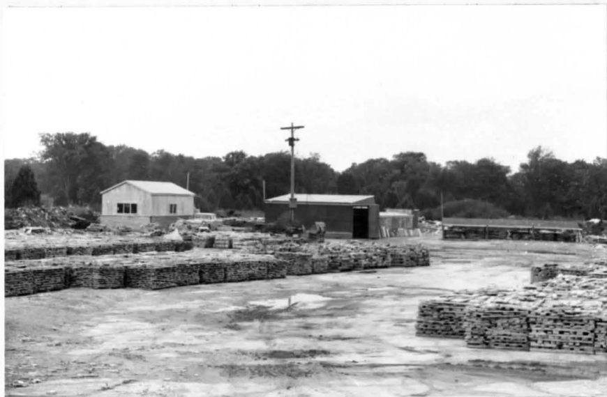
Illus.16 Owen Sound Ledgerock Co. Thin Flat slabs of stone are cut from the bedrock.
