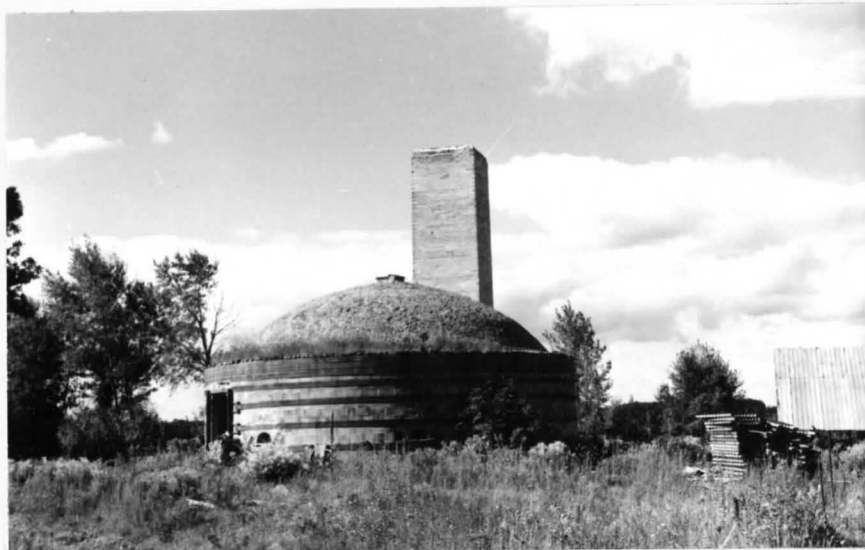
Illus. 8 Such dilapidated structures reveal some of the difficulties which are encountered in the attempt to revive the brick and tile industry.
