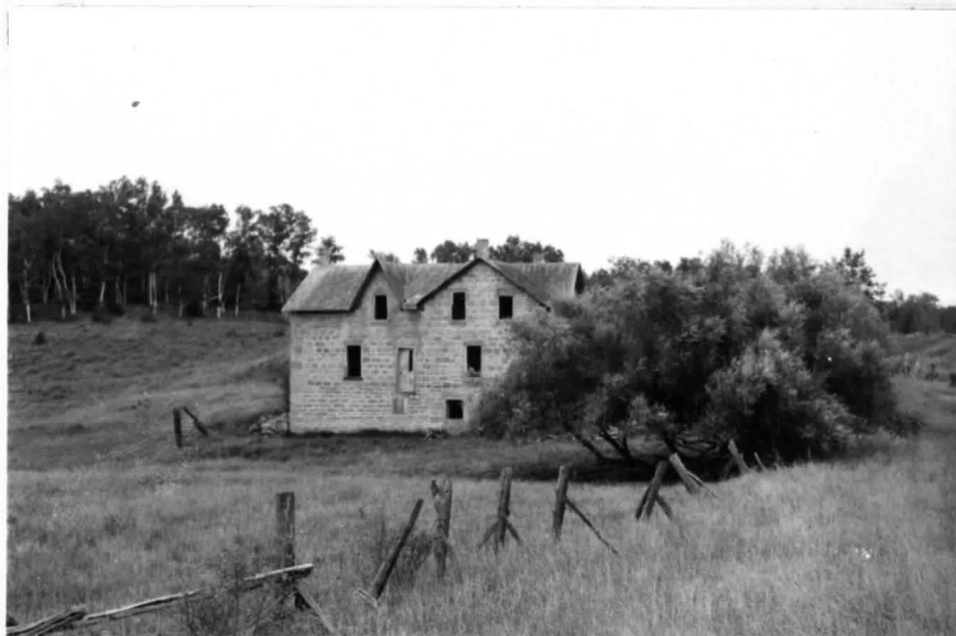
Illus. 10 A large stone farmhouse was an ambitious project, but the land could not support its owners. (Construction material is the local bedrock, the Lockport formation.)
