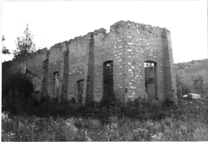
Illus. 7 The shell of one of the buildings of the former Doyle Cement Company at Shallow Lake stands as a monument to the most important industry the township has ever known.
