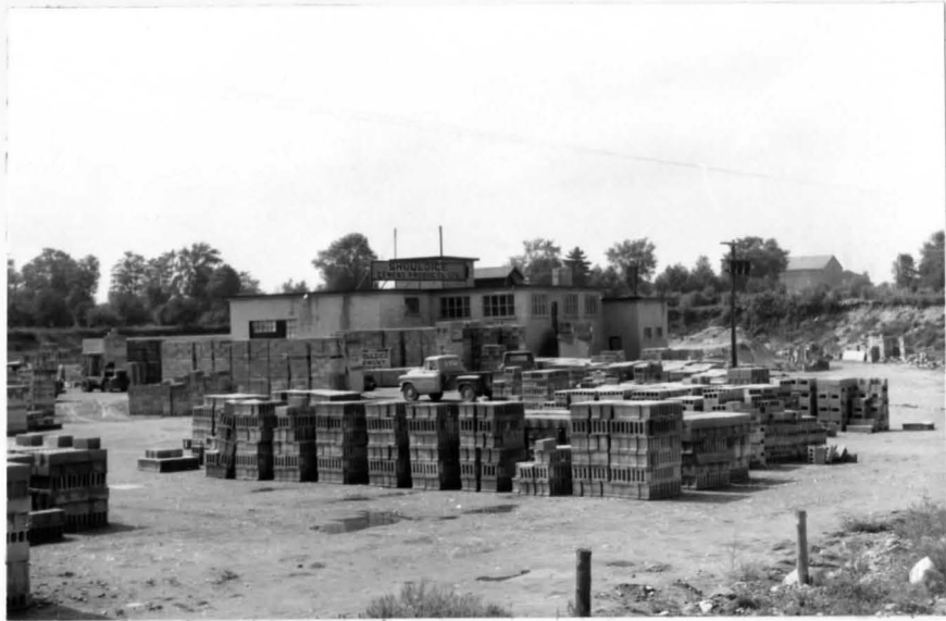
Illus. 15 Shouldice Cement Products Ltd., producing concrete blocks just east of Shallow Lake.
