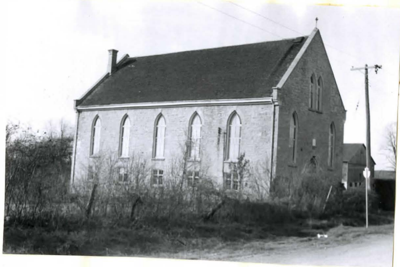
Picture 57. The church at Kirkwall. This church was built in 1848 of limestone quarried in the township.
