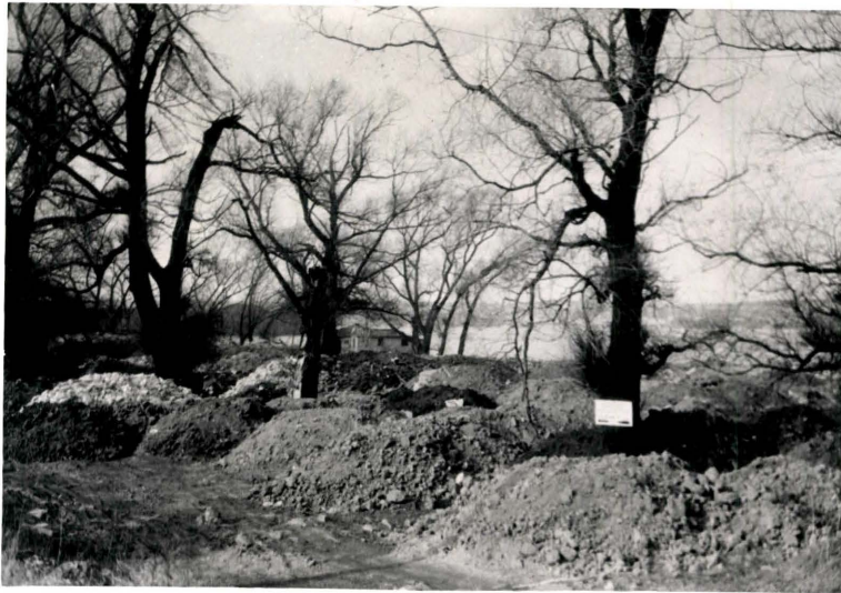
Land reclamation in progress between Wentworth and Hillyard Streets. This part of the Harbour Commission's project north of Ship Street. Sign reads "Dumping garbage prohibited - clean fill only."
