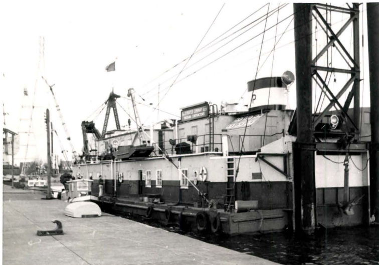
The complicated dredging apparatus owned by J. P. Porter Co., Dredging contractors.
