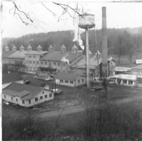
Photo No. 7. The Tillsonburg Borden plant at the intersection of John Pound Street and Borden Crescent. Storage buildings are in the left foreground; heating plant and pump room are at the right.
