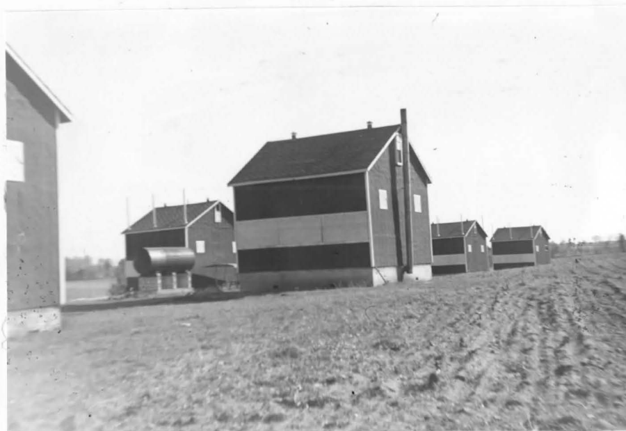
Photo No. 16. A close - up of tobacco kilns with the oil tank at left, used for heating purposes. In the right foreground observe the remnants of tobacco stalks following harvesting operations.
