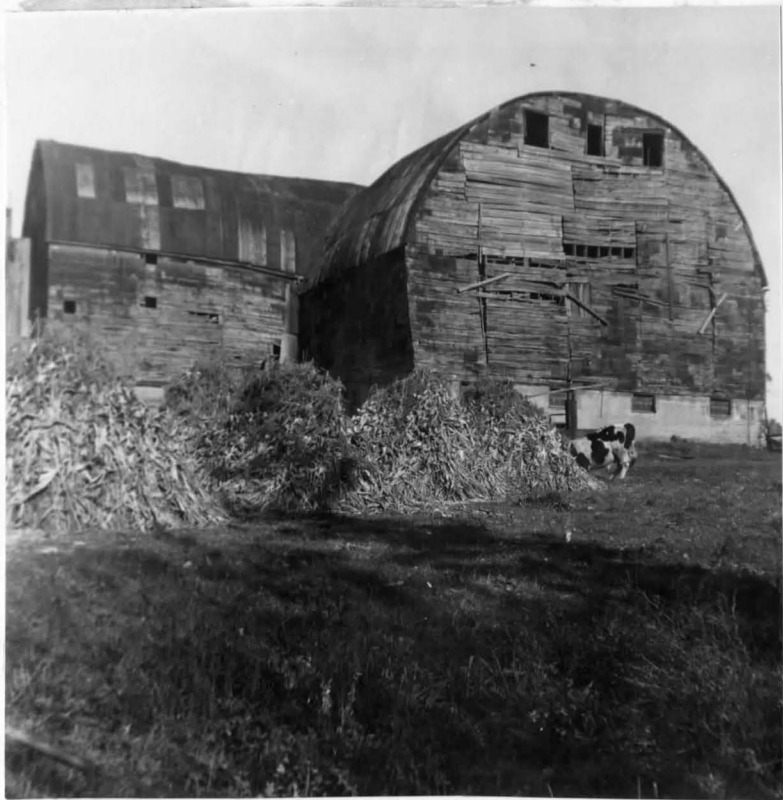
Photo No. 6. A dilapidated old barn located at Culloden.
