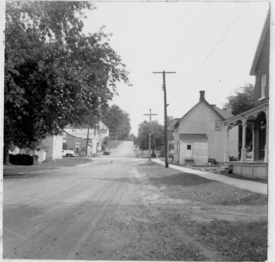
Fig. 5 - 8; A photograph showing the general condition of the streets throughout the residential area.
