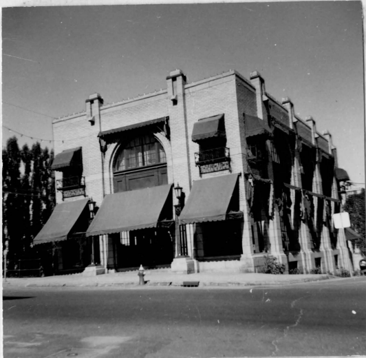
Fig. 4 - 1; Pembroke Electric Light Company, Head office and sub-station..
