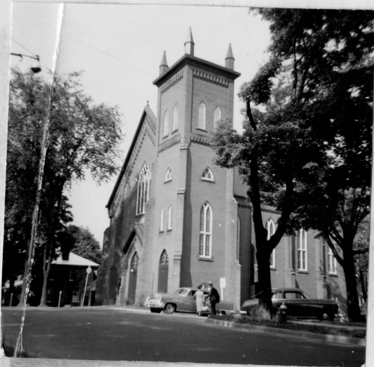
Fig. 5 - 18; Wesley United Church, Pembroke Street at William Street.
