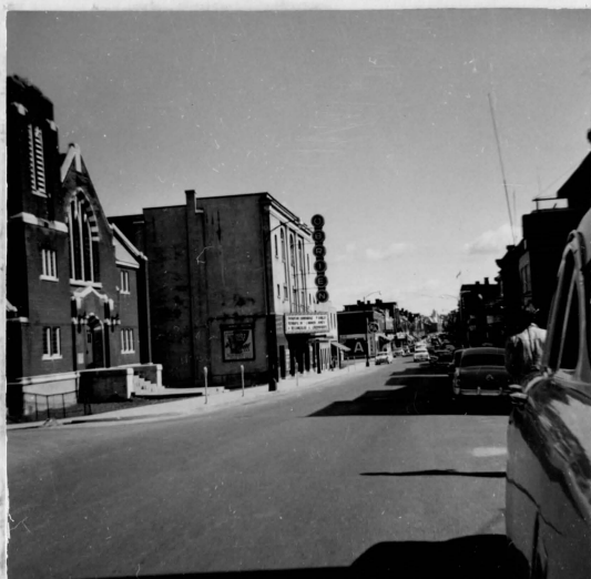
Fig. 5 - 3; The Commercial Core, Pembroke Street looking east.
