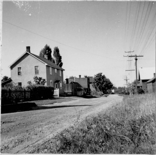
Fig. 5 - 10; 3rd and 4th class housing on Nelson St.
