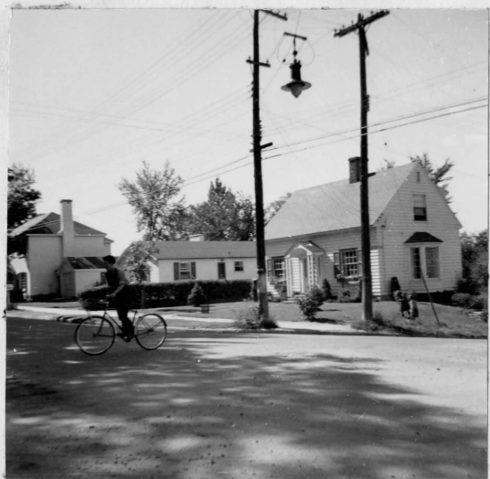
Fig. 5 - 14; 1st class houses on McKay Street (note: railway line runs back of these homes.)
