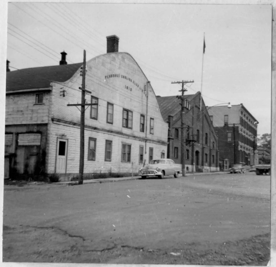
Fig. 5 - 19; Curling rink and armouries, Victoria St.
