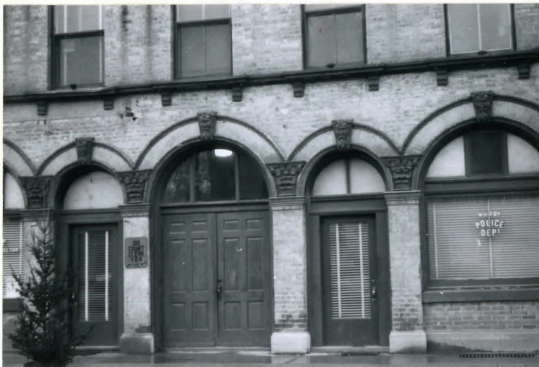
Front of the Whitby Municipal Offices.
