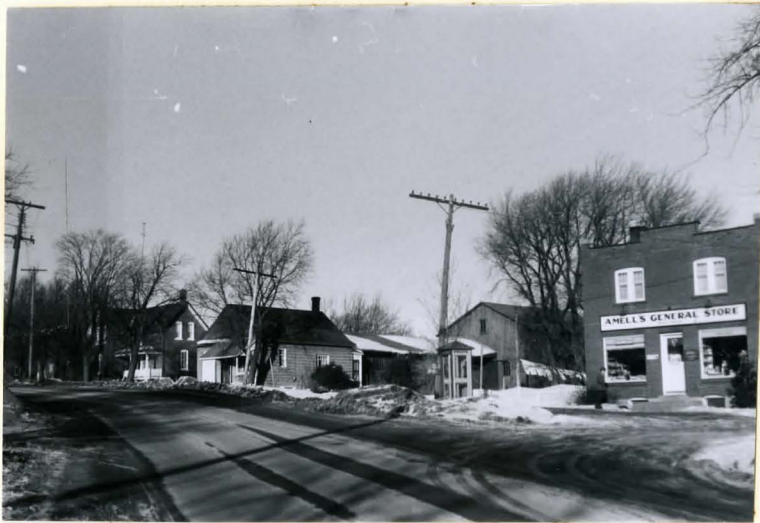
The hamlet of Myrtle Station looking north from the Station.
