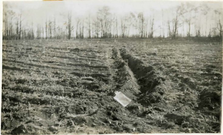
FIG 17. Drainage ditch in the Lincoln-Caistor Clay plain. Size of lecture board approximately 10" x 12".
