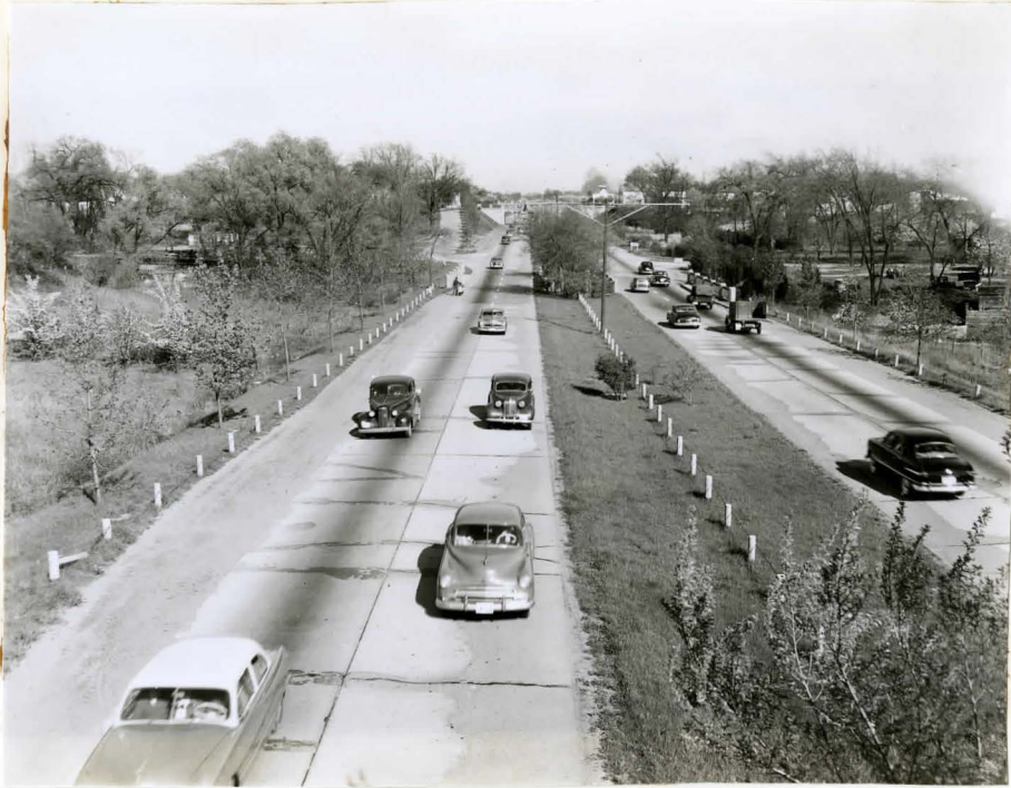
FIG 9. Queen Elizabeth highway. Note the heavy traffic.
