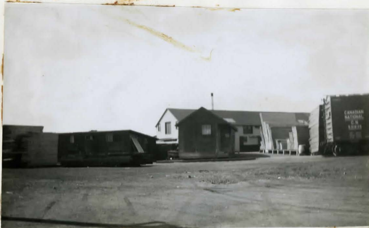
FIG 22 A lumber yard on the Canadian National Railway main line.
