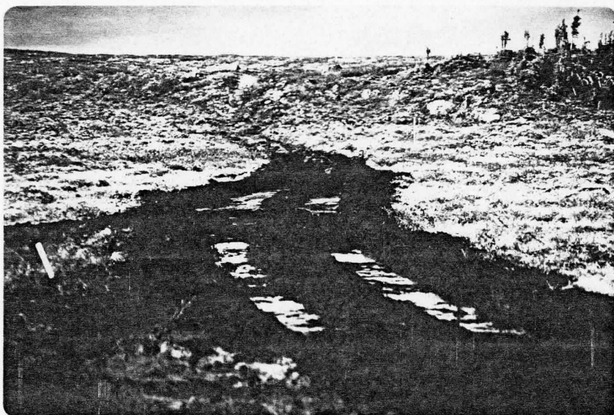
Figure 4.10 The north-south section of main track 1 showing the susceptibility of peat (foreground) and till (background) to disturbance.
