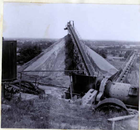
Number 10. Large quantities of sand and gravel for the building trades are extracted from the glacial delta. This pit is rapidly expanding at the expense of neighbouring orchards.
