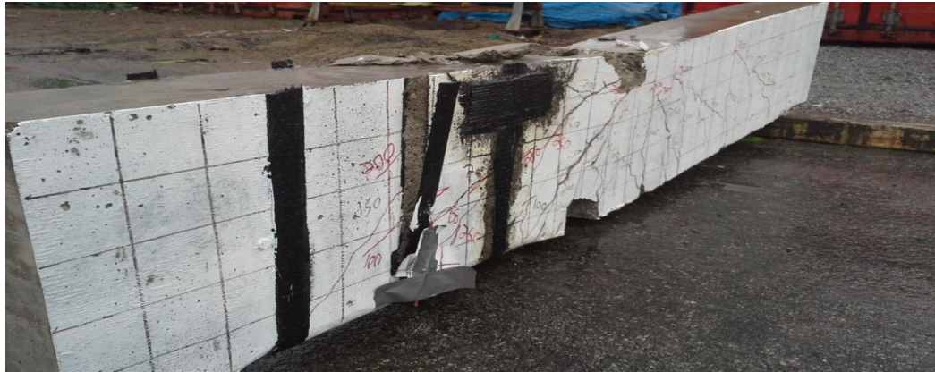
Figure 4-37: Image of beam U-45-H-1L at failure
