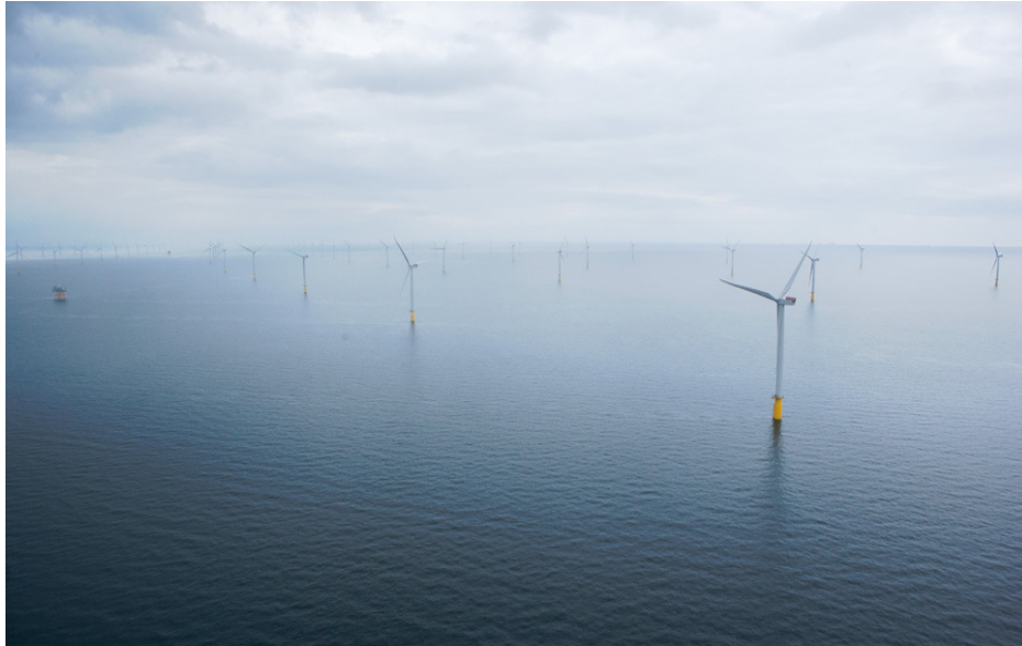
Fig. 3.1. Walney off-shore wind farm [2].
