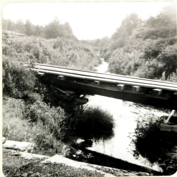
photo. 15 : A view of one of the drainage ditches installed to lower Welland Bog's watertable so that extension of agriculture might be feasible. The narrow gauge railway in the foreground is used to convey peat moss from the bog to a local processing plant.
