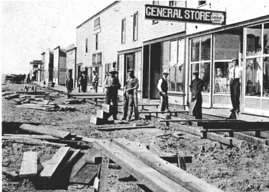
Robsart's wooden sidewalk construction, 1914
