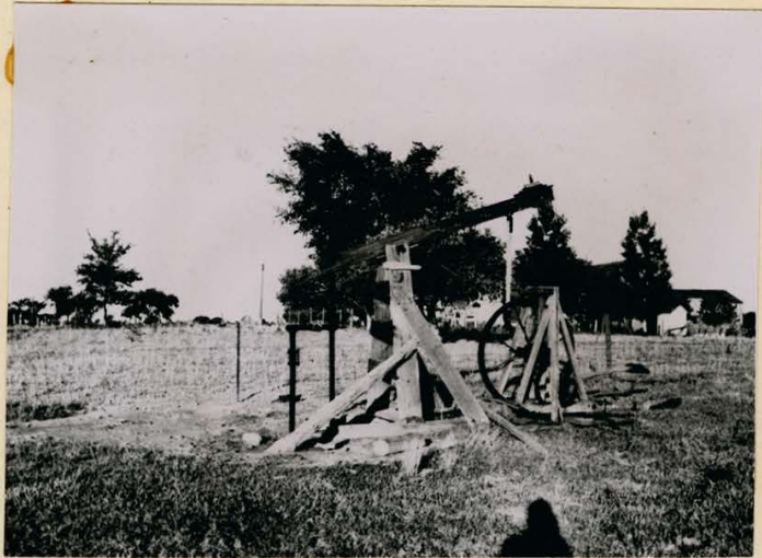
An old gas well near York. This well has to be pumped out periodically because pressure is very slight.
