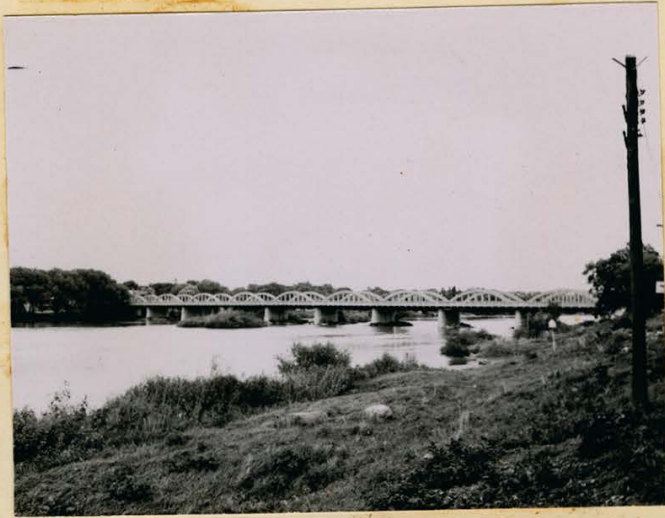
The concrete bridge at Caledonia which carries the heavy traffic of Highway No. 6.
