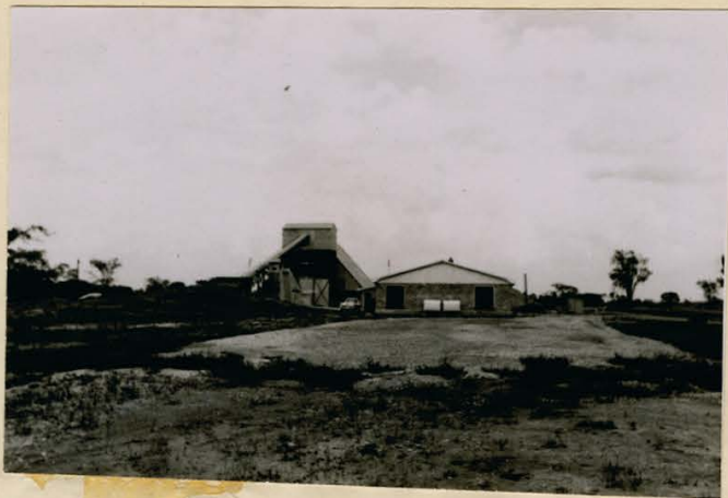
The head of the G.L.A. mine, one mile west of Highway No. 6.
