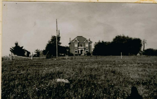
An old farm house on Highway No. 56 being used as a suburban residence. The land is being used as pasture for beef cattle.
