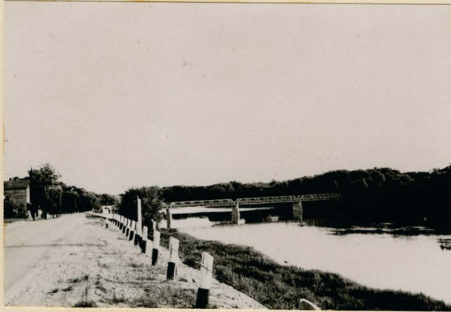
The bridge at York which carries only a small amount of local traffic.
