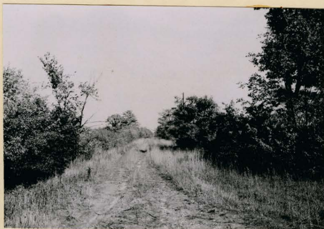
A road in the eastern end of the Township which is used only for farm machinery. For much of the year it is impassible.
