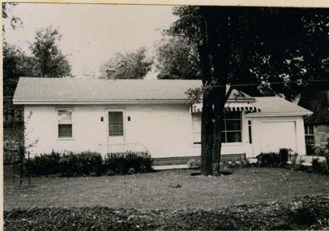
A new fourth class home on the south bank of the River. This is smaller than most of the older fourth class homes.
