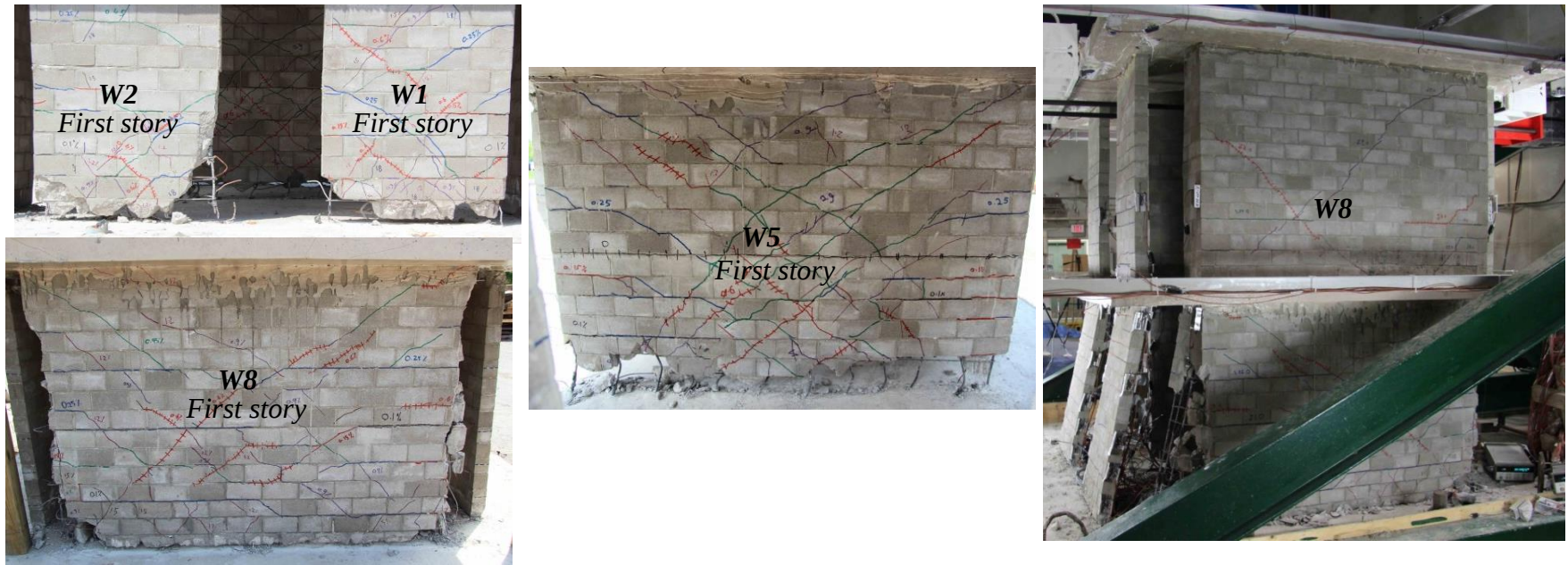
Fig. 4.9: Sliding failure at the end of the test.
