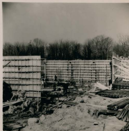
Fig. 10-4 Boiler House Concrete Forms 27-4-70
