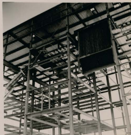
Fig. 10-12 Air Preheater Installation 7-7-70
