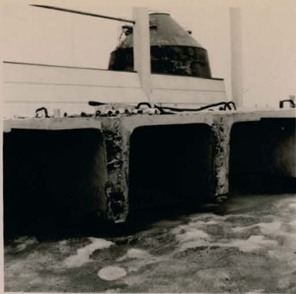
Fig. 10-37 Typical Receiving Bldg. Roof Beam 21-2-71
