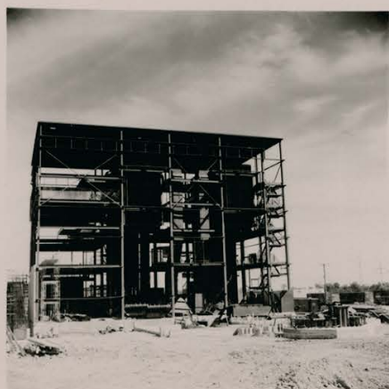
Fig. 10-23 View LN Boiler Erection nearing finish 12-9-70
