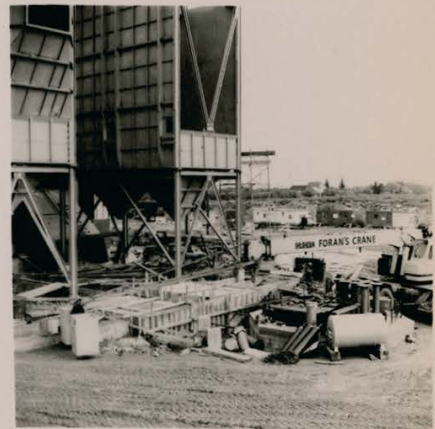
Fig. 10-27 LN Two Views of Precipitator Shells. Note stack foundation in foreground. 1-11-70
