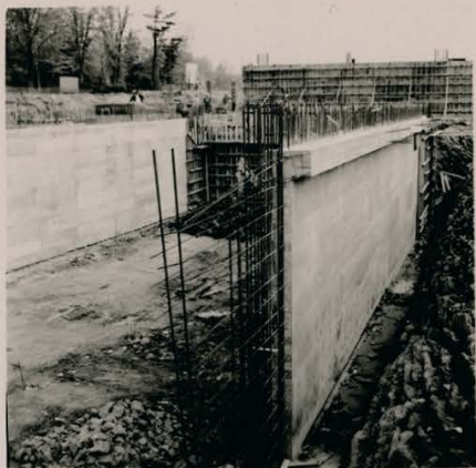
Fig. 10-7 Receiving Pit Walls 27-5-70
