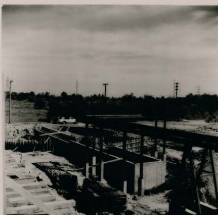
Fig. 10-21 Steel racks for ash handling system. Silo foundation in back 12-9-70
