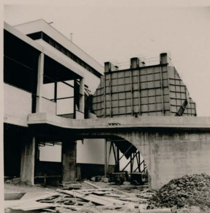
Fig. 10-41 Entrance Ramp, Precipitator, LE 17-4-71
