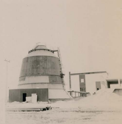
Fig. 10-42 Silo, Exit Ramp LS 17-4-71
