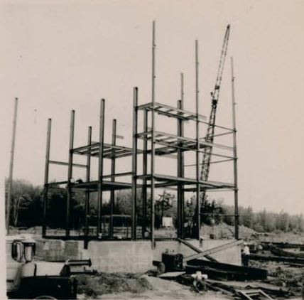
Fig. 10-8 Boiler House Steel Erection 27-5-70
