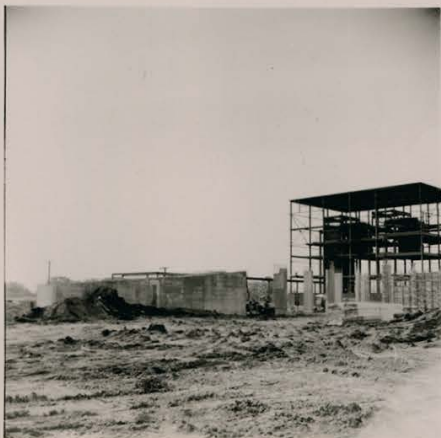
Fig. 10-17 View LS Note exit ramp 23-7-70
