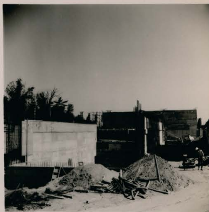
Fig. 10-16 Receiving Pit LN 21-7-70
