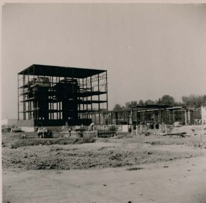
Fig. 10-19 View LS Note exit ramp and ash- handling steel 11-8-70
