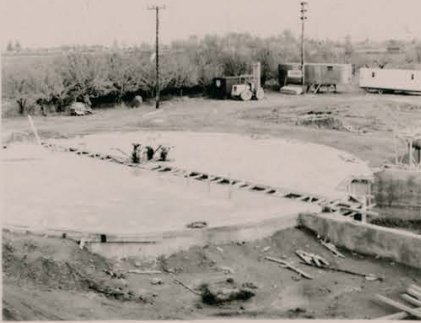
Fig. 10-25 Base for Atlas Silo, looking NE Note trench 1-11-70
