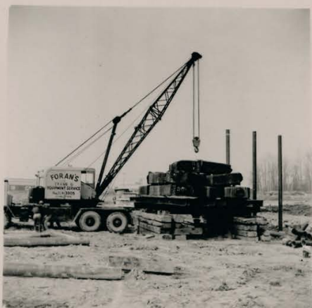
Fig. 10-5 Pile Relaxation Testing (200 tons) 27-4-70
