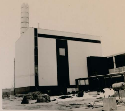
Fig. 10-38 Boiler House LS 21-2-71
