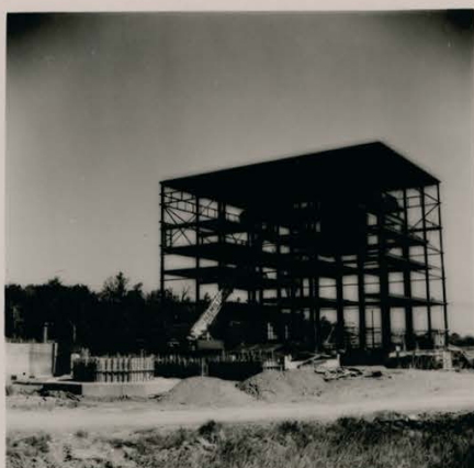
Fig. 10-9 Boiler House LN 7-7-70
