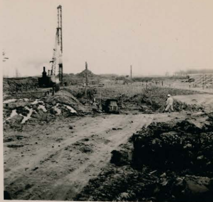
Fig. 10-2 Pile Driving at Receiving Pit 27-4-70
