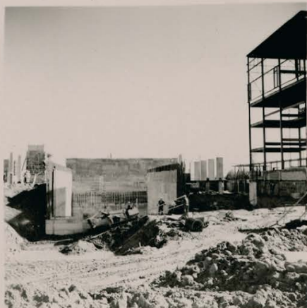
Fig. 10-11 Backfilling Receiving Pit 7-7-70
