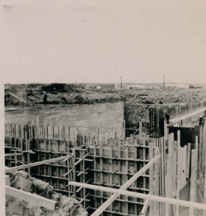
Fig. 10-6 Receiving Pit Concrete Forms 27-5-70
