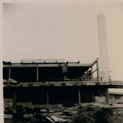
Fig. 10-40 Office Area, Rec. Bldg. LE 17-4-71
