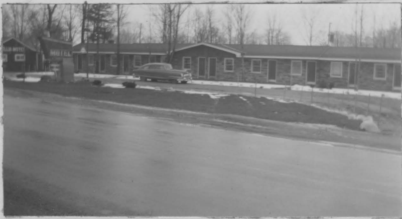
MOTEL DEVELOPMENT ON HIGHWAY NORTH OF ORILLIA
