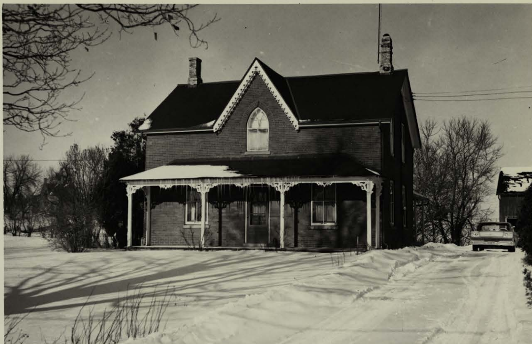
A Gothic Revival-style stone home, characteristic of the Middle II Period in Township of Puslinch.
