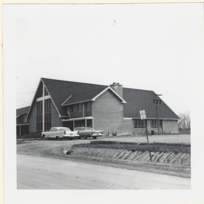
Fig. 11 Thornhill United Church. This new building is representative of the growth in institutional construction that is proceeding.
