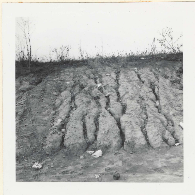
Fig. 4 Erosion on a road-side embankment. This is not common on the grass-covered fields. Note size of rills in relation to cigarette package in the centre.
