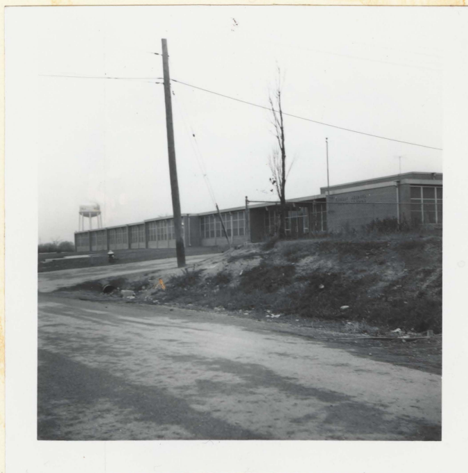
Fig. 23 A public school in Richmond Hill near new homes and the industrial section. The new water storage tower appears in the background.
