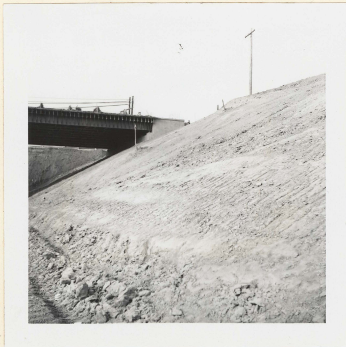
Fig. 3 A new road cut shows the stone-free clay parent material and soil that is characteristic of most of the area.
