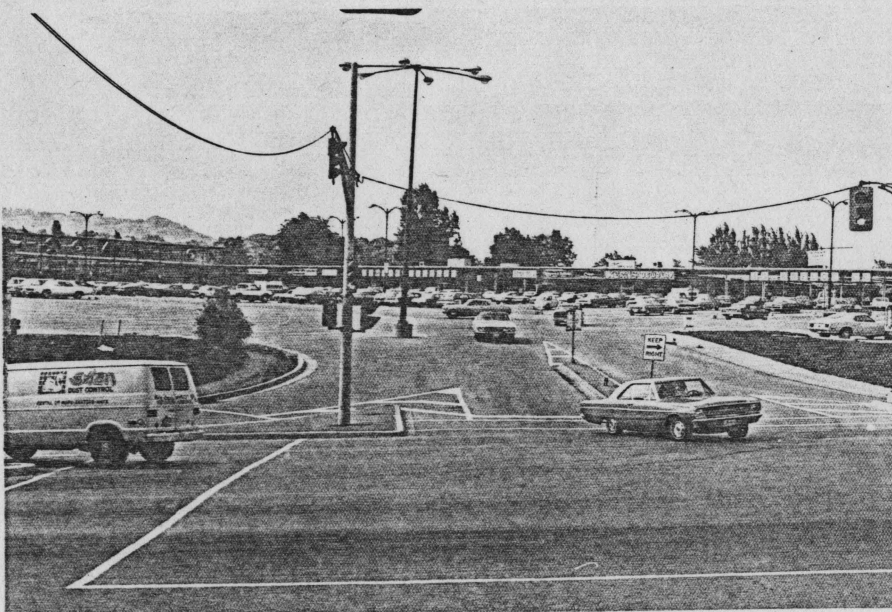
(a) Looking south from the intersection with Grant Blvd., the major axis with its lack of adequate signing and barriers creates a hazardous situation for motorists.
