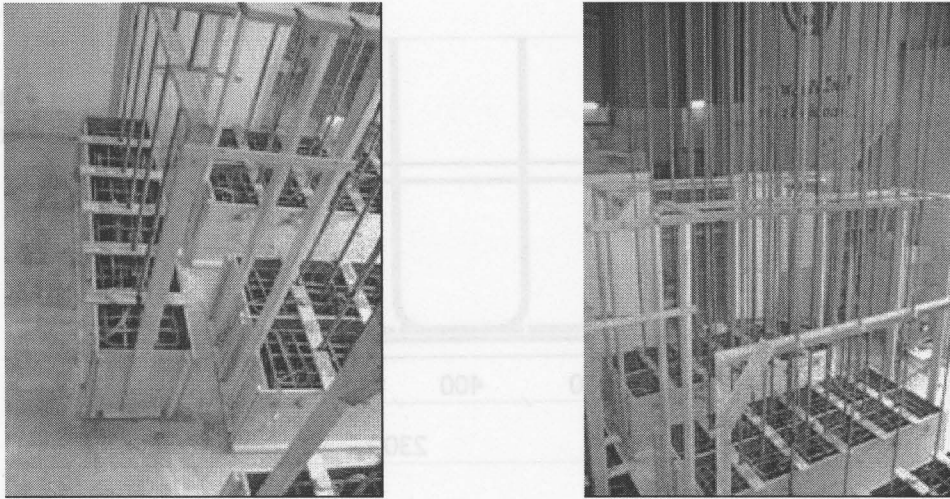
Fig. 2. 4: Temporary support of vertical steel during concreting of base beam
