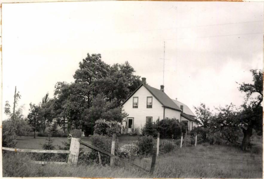
A typical second class farmhouse found in the areas of general farming. Note frame construction, neat and tidy appearance.
