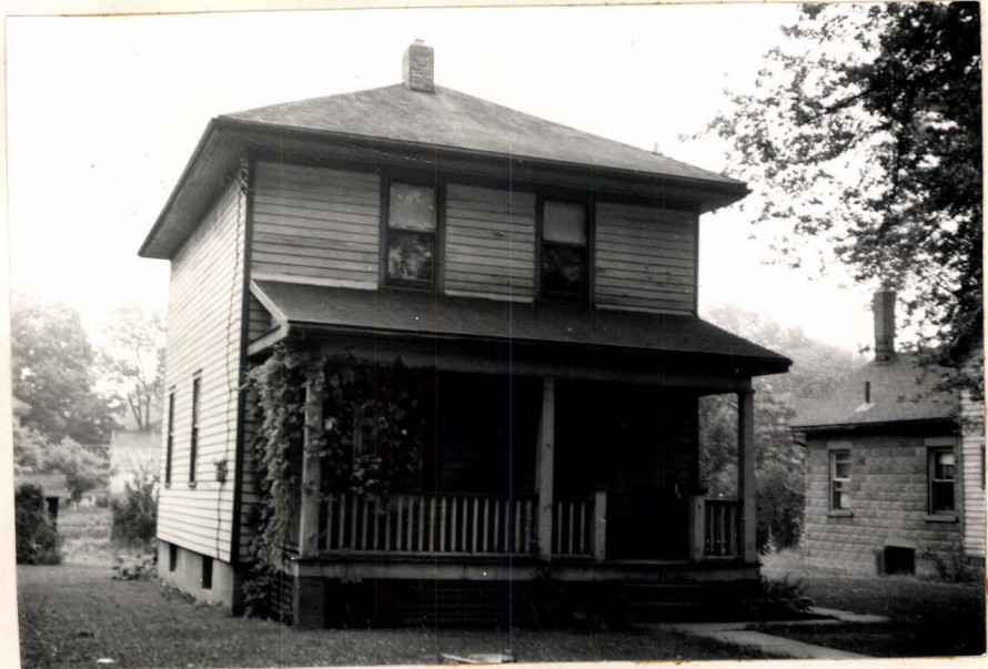
An example of Fourth Class housing in Port Dover. Note dirty, untidy appearance, and lack of paint.
