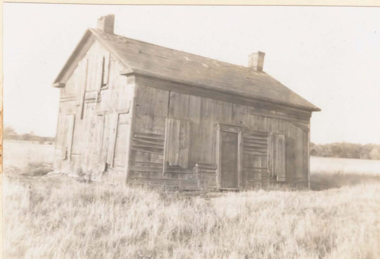
14. An example of farm amalgamation. This house has been abandoned and the land amalgamated into another holding.
