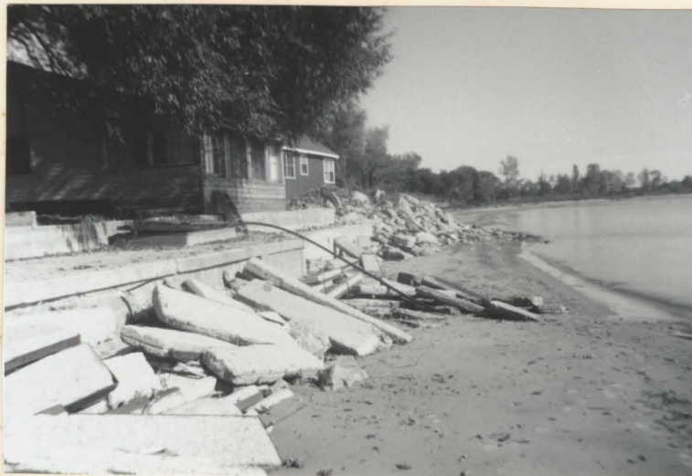
29. A make-shift breakfront at Woodlawn Park. There is no bank here and the breakfront has been built to protect the buildings from wave action.
