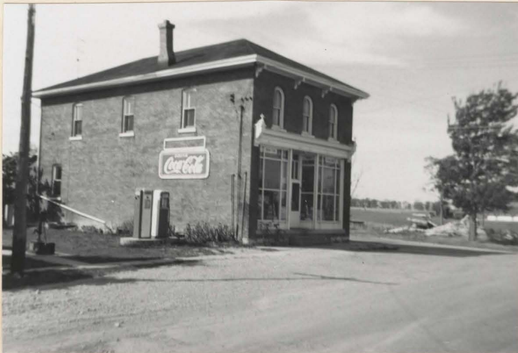
• The general store at Cheapside. This is typical of such stores throughout the study area.
