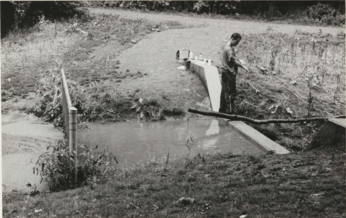
Figure A1.3 The stormwater detention pond's dam late in the August 7/86 storm event. Water is backing up behind the dam reducing water velocity.
