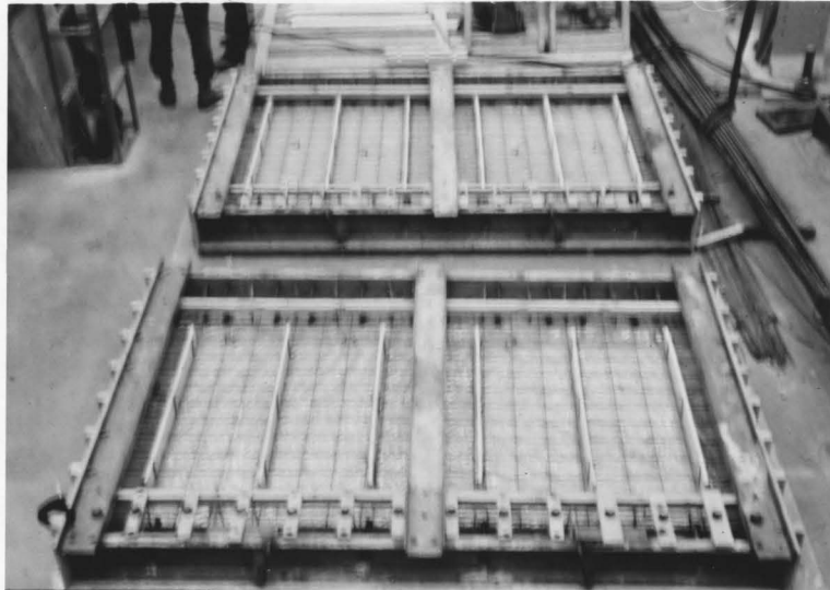
Fig. 18 PANELS C AND D READY FOR POURING
