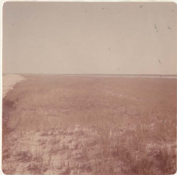
Fig. 2:13 General View of defunct inlet on North Beach.
