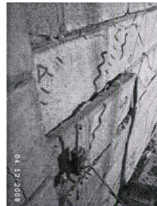
c) Bulging of face shells
