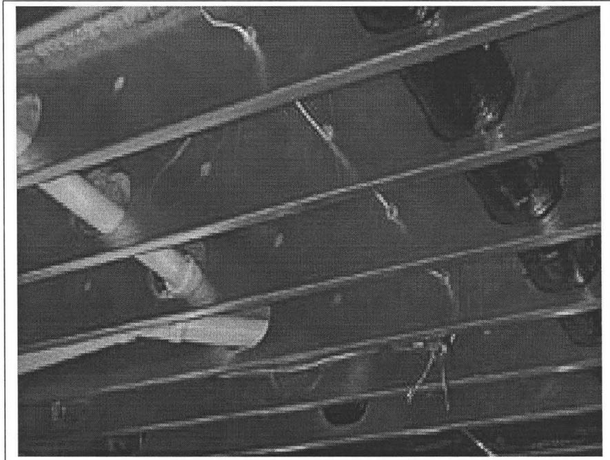
Figure 1.5: Application of web openings in cold-formed steel (CFS) joists (<http://www.aegismetalframing.com>)
