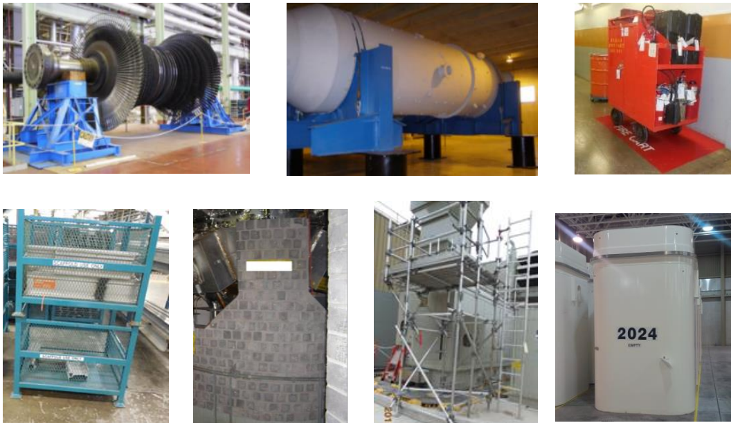
Figure 1-1: Examples of unanchored objects that are vulnerable to rocking and overturning inside a NPP. (Clockwise from top left: idle turbine rotor, vessel in storage, hand cart, dry storage container (fuel cask), scaffold, radiation protection masonry, storage bin. (Photo courtesy: Bruce Power, and Western Used Fuel Dry Storage Facility (Ontario Power Generation), Ontario, Canada)
