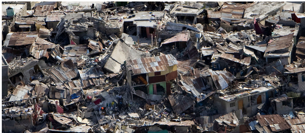
Figure 6.15: An aerial photograph taken in 2010 depicting the devastation and collapse of infrastructure caused by the earthquake in Haiti.
