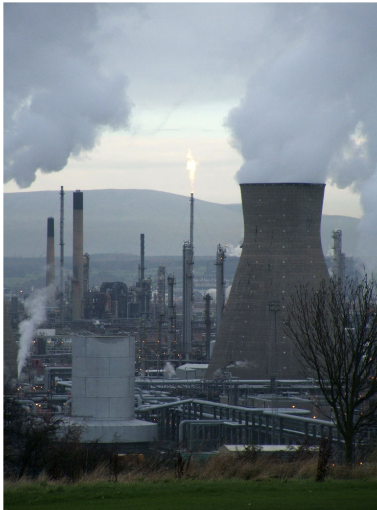
Figure 5.8: A petrochemical refinery found in Grangemouth, Scotland, UK. At refineries like these, petroleum is separated using distillation into its component parts: many different important chemicals, including acetone, benzene, naphthas, and gasoline are produced at plants like these.
